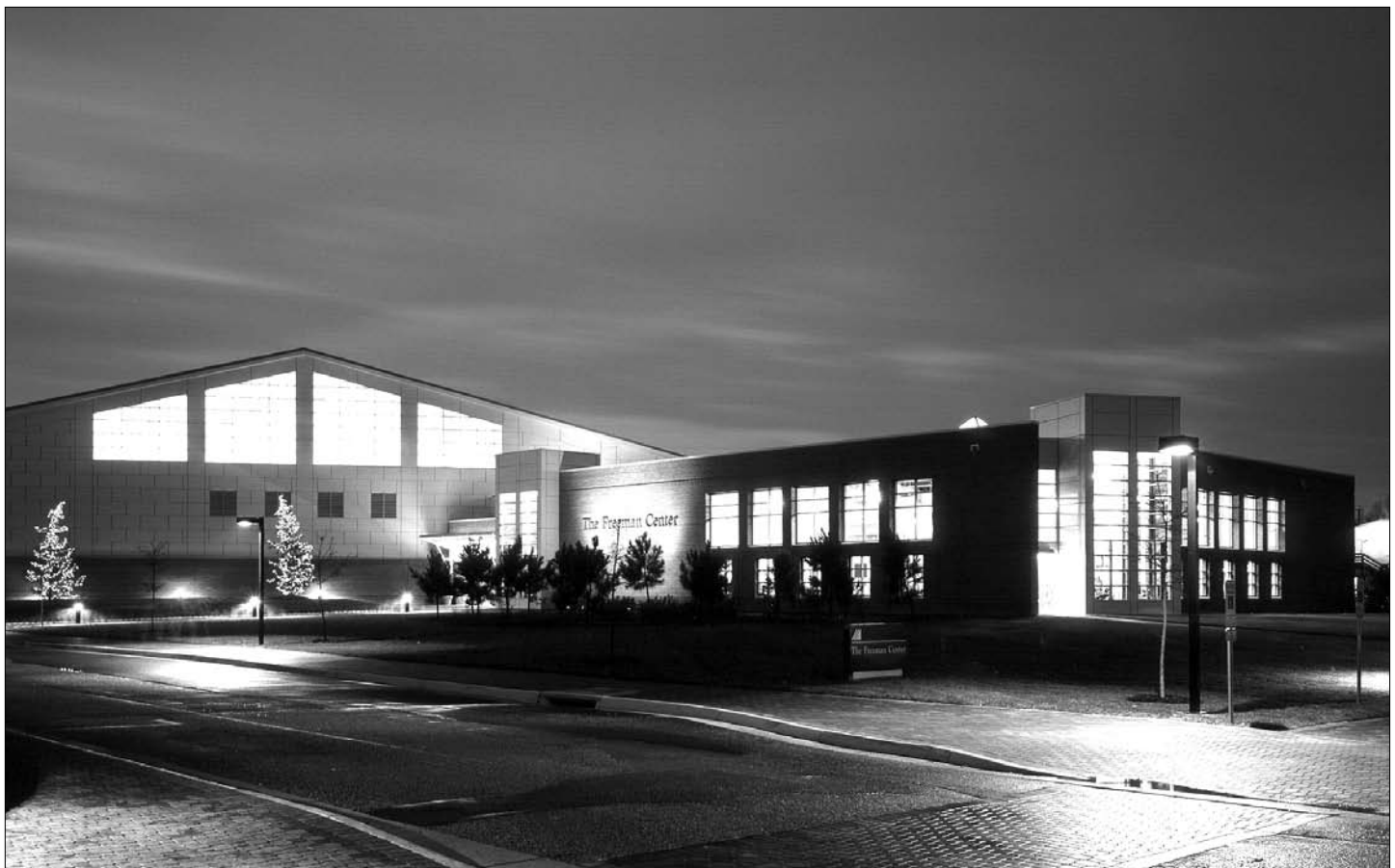
The Freeman Center at night
